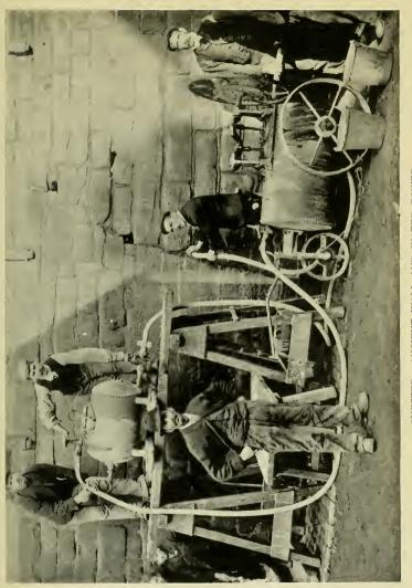
CHESTER, ANCIENT WALL AND WATER TOWER. The Greathead grouting machine being applied for the first time in the saving of ancient buildings.
